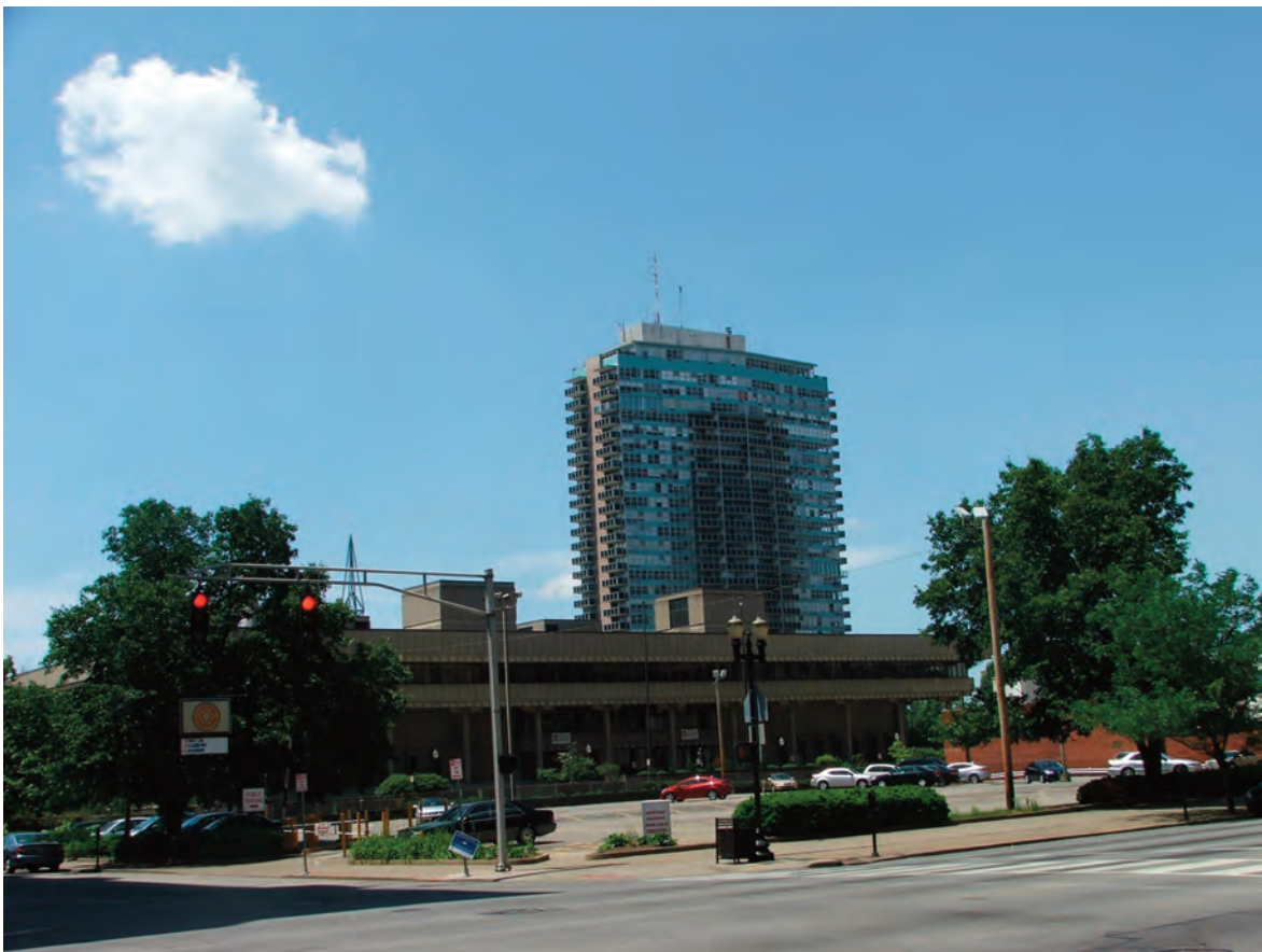
View of Museum building site from northeast corner of Broadway and Third Street with library and 800 Building in the background.
