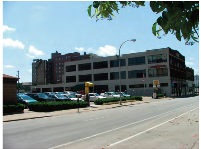
View from southern edge of museum site to Park and Luckett Farley building
